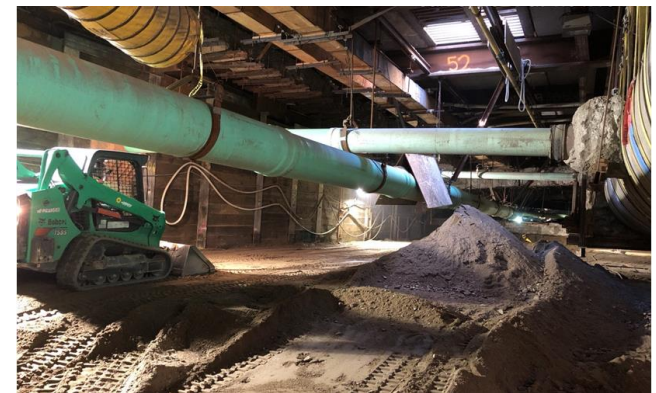
Backfill operations above roof slab at Flower St
