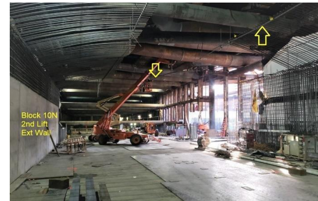
Installing Roof Rebar at Wilshire/Fairfax
