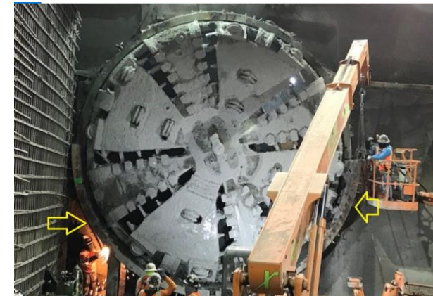
Purple TBM Arrival of Wilshire/La Cienega Station
