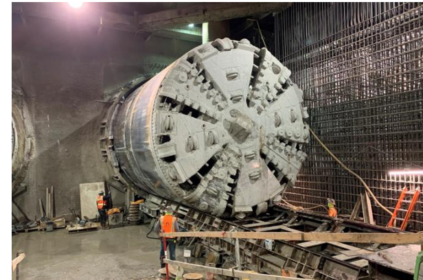
Red TBM Arrival of Wilshire/La Cienega Station
