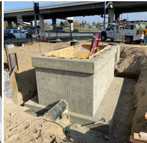
Formed & poured North Drainage System
