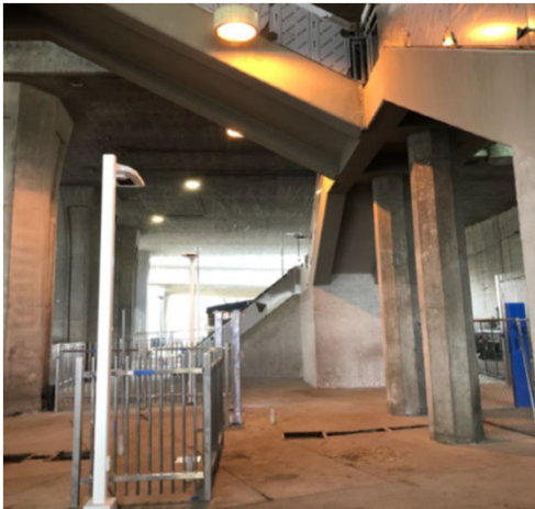
Completed concrete work @ C Line west
