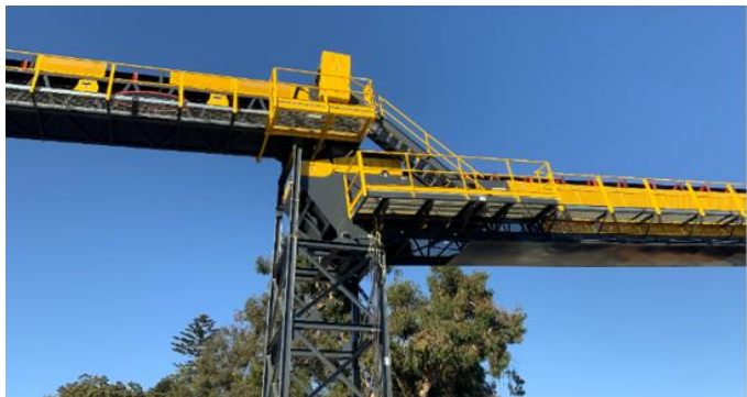
Conveyor Belt Assembly for TBM Operation at Tail Track Exit Shaft
