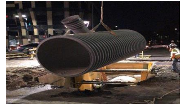
Sewer Relocation for Westwood/UCLA Station
