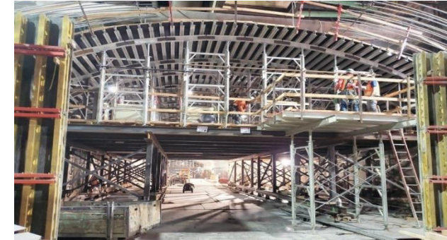
Roof Falsework Installation at Wilshire/Fairfax Station
