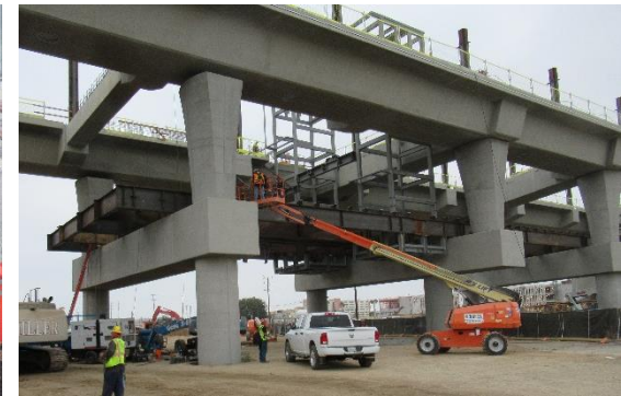
LAVA APM Steel Work in Progress
