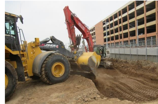
On Site Backfilling Work
