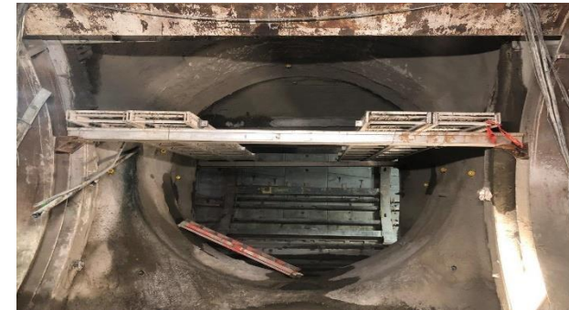
Excavation Complete at Cross Passage #16 (Reach 2)
