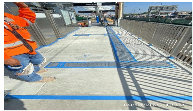
Hyde Park – Preparing the floor surface at the south end entrance ramp for coat finish placement
