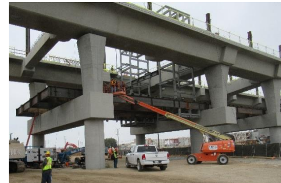
LAVA APM Steel Work in Progress
