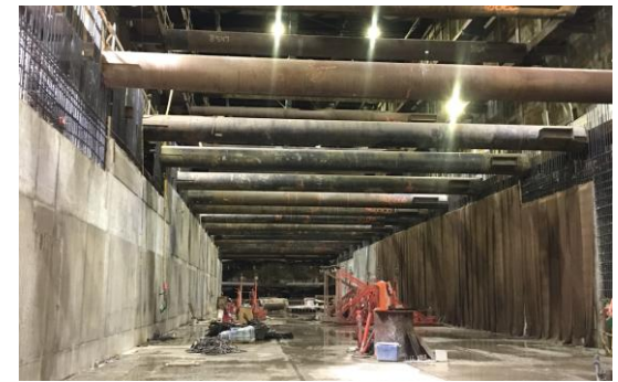
First Level Walls at Wilshire/Rodeo Station
