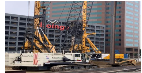
SOE Pile Installation for Westwood/UCLA Station
