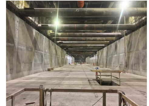
First Level Walls at Wilshire/Rodeo Station
