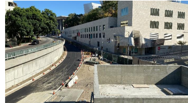
Concrete curb & gutter at 2nd Place/Flower
