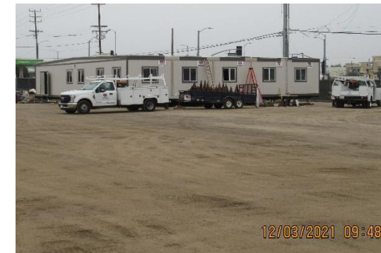
Mobilization for Main Station Construction
