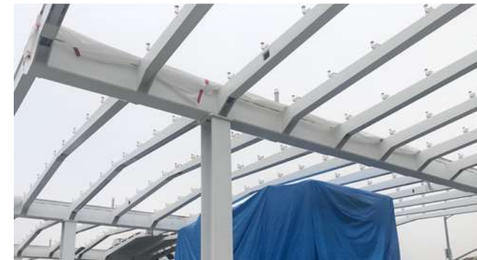
Little Tokyo/Arts District Station Canopy Installation
