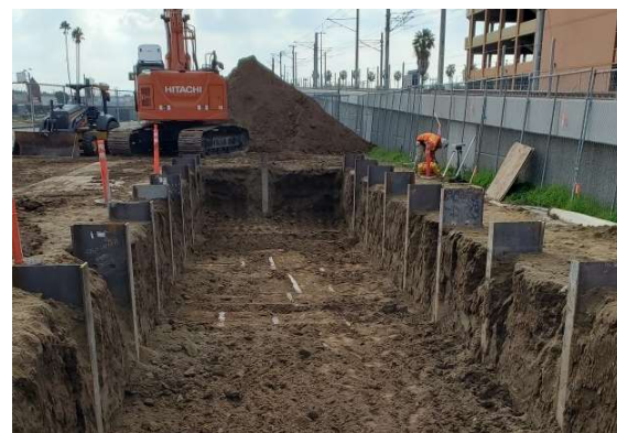
Shoring in progress
