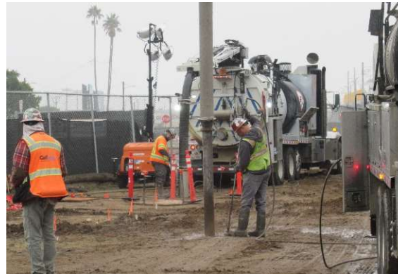
Shoring installation for Stormwater System
