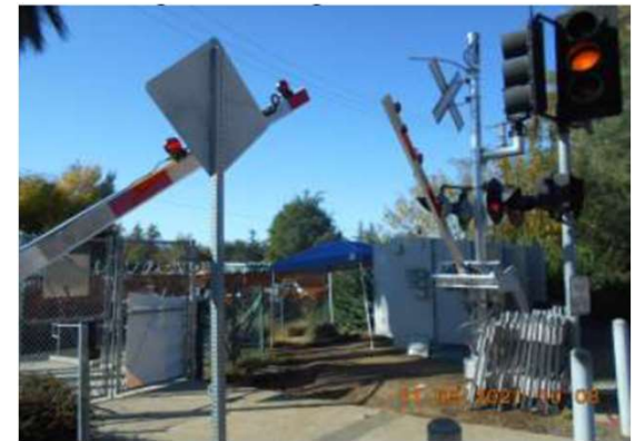
Pilot Gate - Testing
