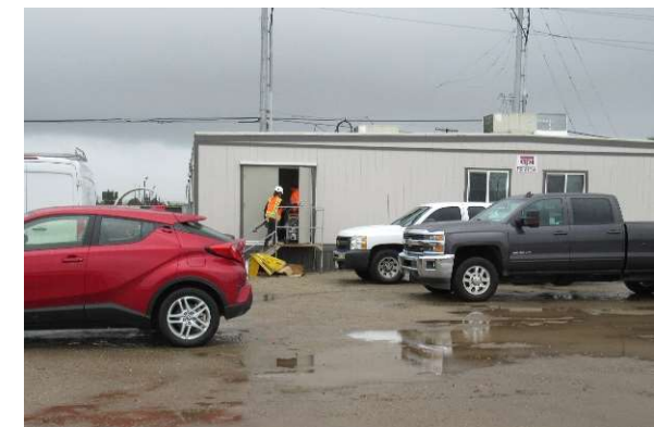
Mobilization for Main Station Construction
