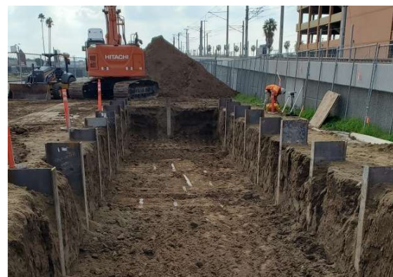
Shoring in progress
