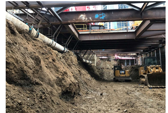
Constellation Station Entrance Excavation
