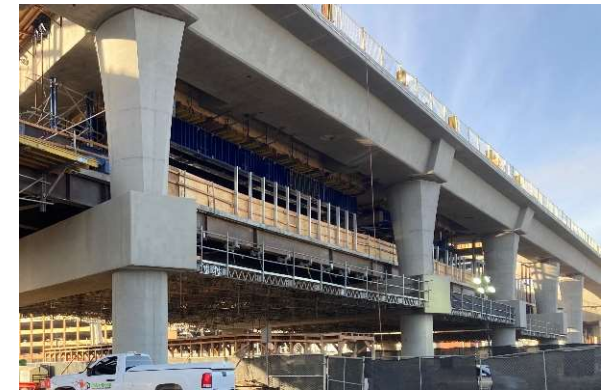
LAWA Station work in progress
