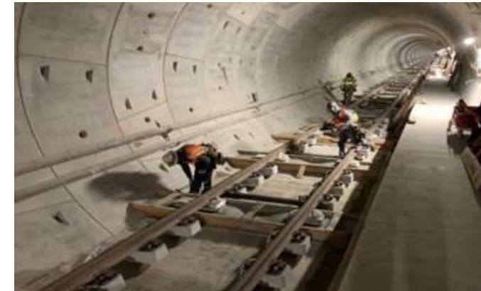
Reach 1 North Tunnel Trackwork Installation
