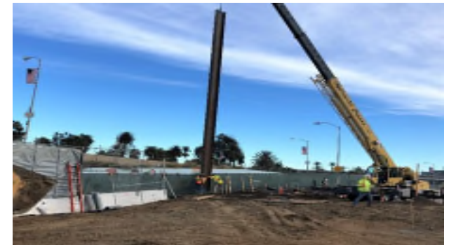
SOE Pile Installation for VA Steam Tunnel Relocation
