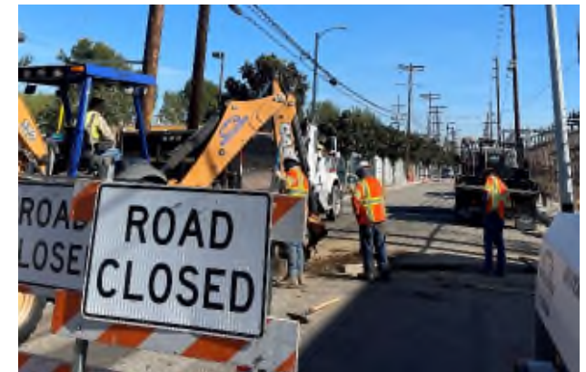
DWP Sylmar Undergrounding
