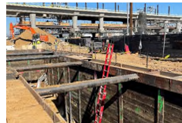
Shoring near completion for east cistern
