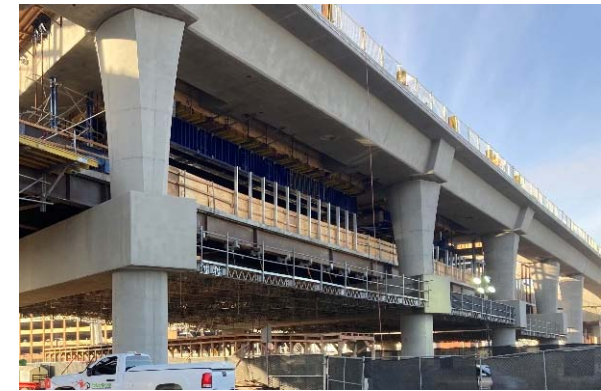
LAWA Station work in progress
