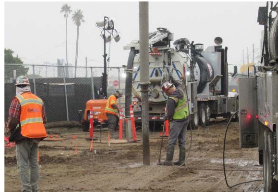
Shoring installation for Stormwater System
