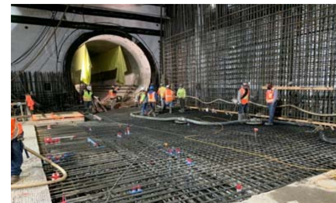
Concrete Placement at Wilshire/La Cienega Station (West)
