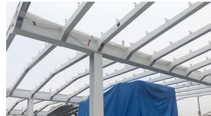
Little Tokyo/Arts District Station Canopy Installation
