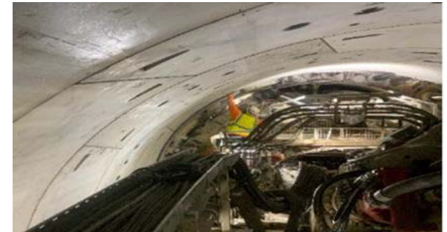
Ring Installation in the BL Tunnel
