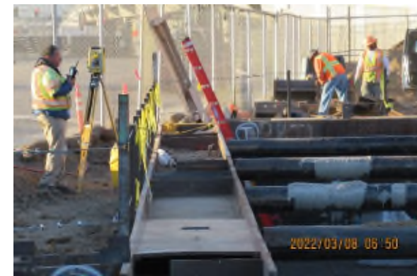
East cistern work
