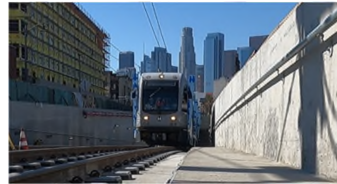
Light Rail Vehicle operated under its own power
