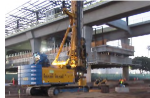
CIDH pile work near APM Station
