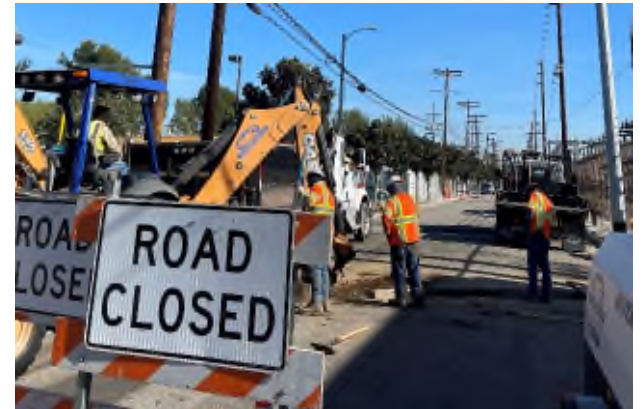
DWP Sylmar Undergrounding
