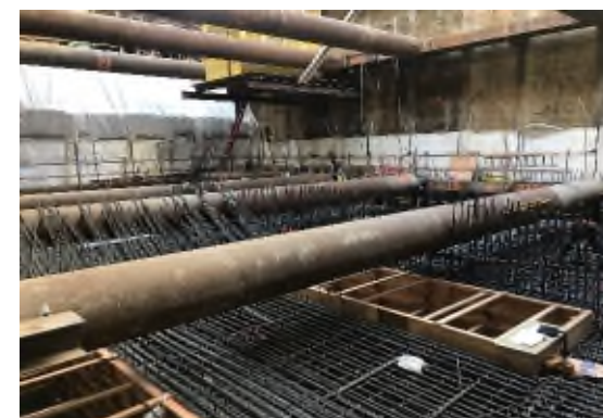
Rebar Installation at Wilshire/Rodeo Station Entrance
