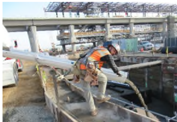
Backfill at cisterns
