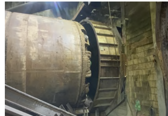
Harriet Break-out at Wilshire/Rodeo Station
