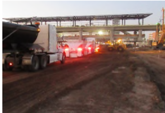
Early morning soil removal work
