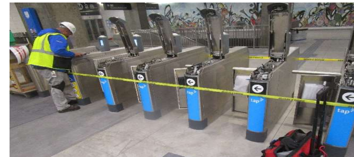
MLK Station – Performing configuration programming and software testing to TVM and fare gate system
