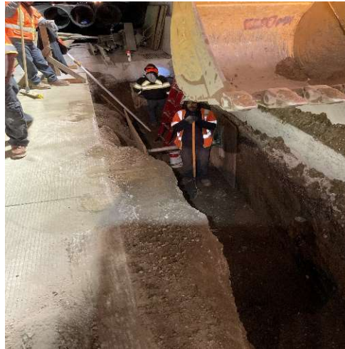
Drainage excavation on SB I-5 median DS# 159
