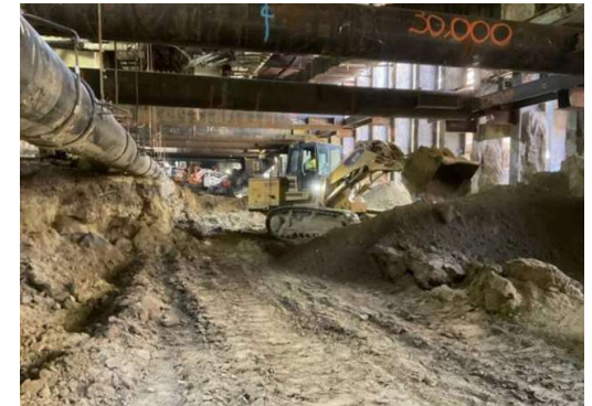
Century City Constellation Station Box Excavation
