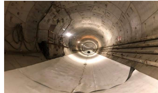
Layout HDPE in Reach 2 Tunnel
