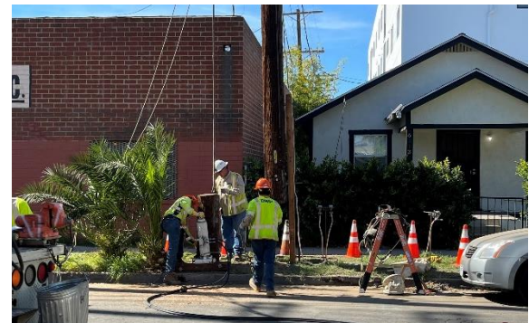
DWP Vesper Advanced Utility Relocation
