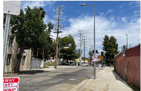
DWP Overhead Construction at Vesper
