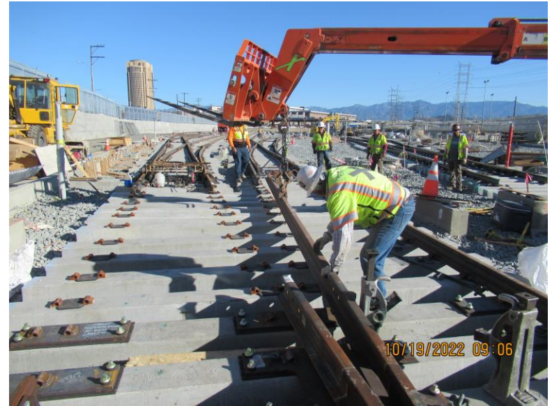
North Yard Storage Tracks
