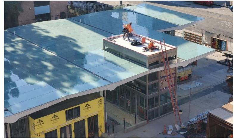
Installation of TPO roofing (Historic Broadway Station)
