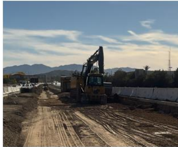
On-Going Roadway Excavation in the Median
