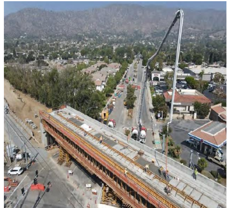
Foothill Grand - LRT ductbank walkway
