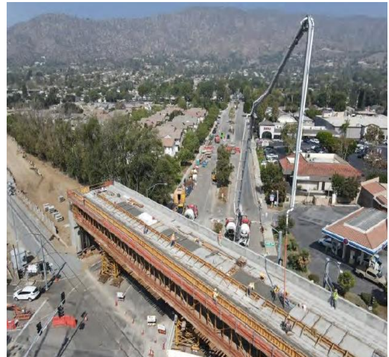
Foothill Grand - LRT ductbank walkway
