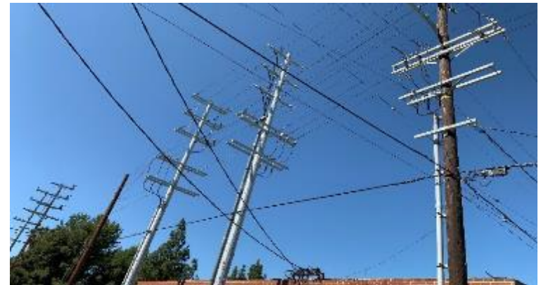
DWP Overhead Construction at Vesper
