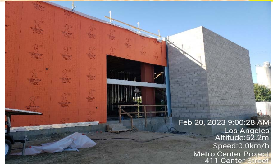
Exterior Finish – Weather Barrier & Sheet Metal
