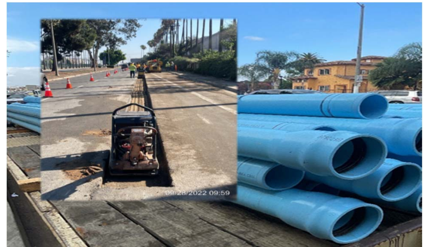
Preparing & Installation of PVC pipe at Florence between Prairie/High Street
