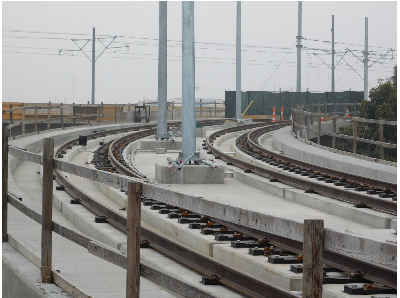
Crenshaw project – K Line – elevated tracks
