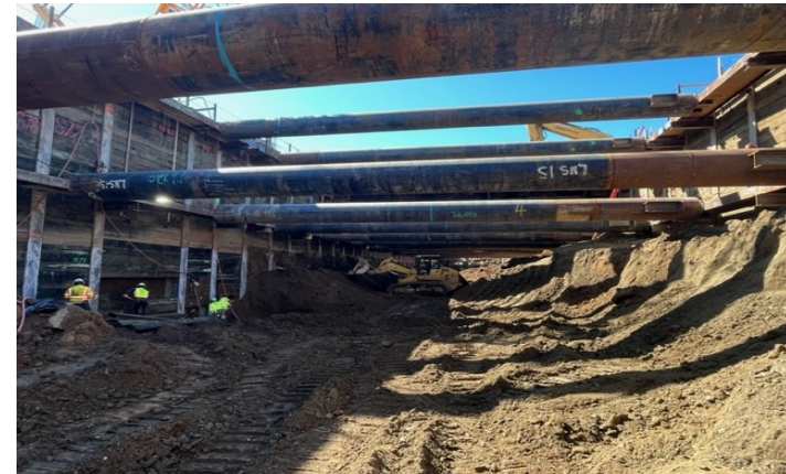
Westwood/VA Station: Excavating station for Level 2 Bracing
