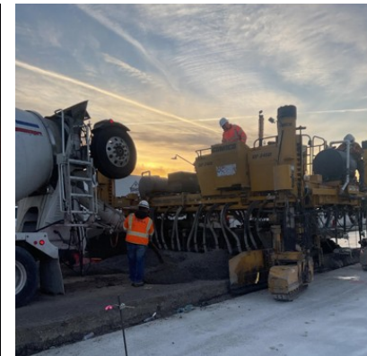
Paving Lean Concrete Base (LCB) in the Median On-Going
