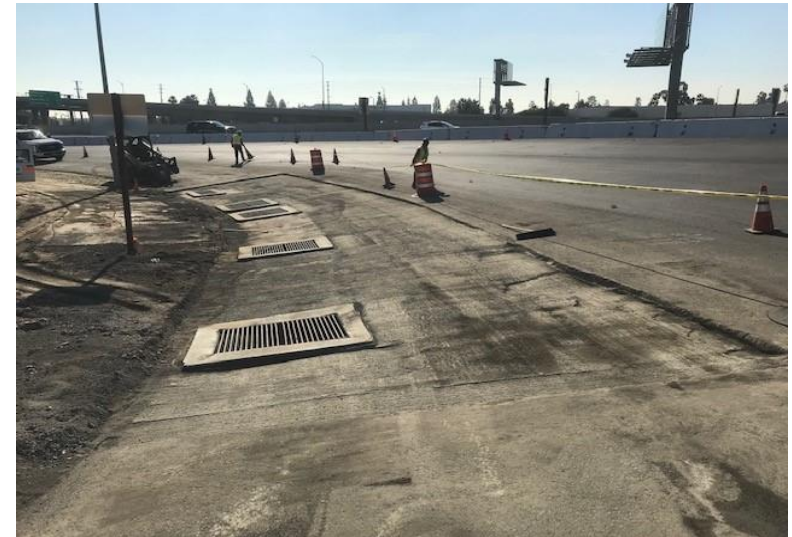
Northbound Valley View offramp
