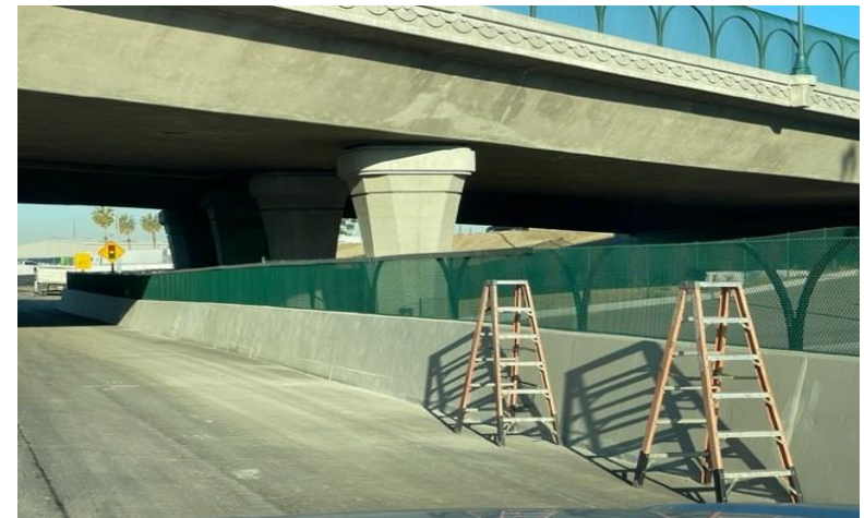
Finalizing fence on barrier
