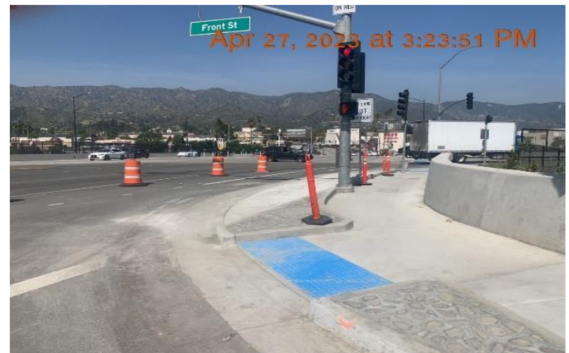
Bike lane improvement at Burbank Blvd overcrossing
