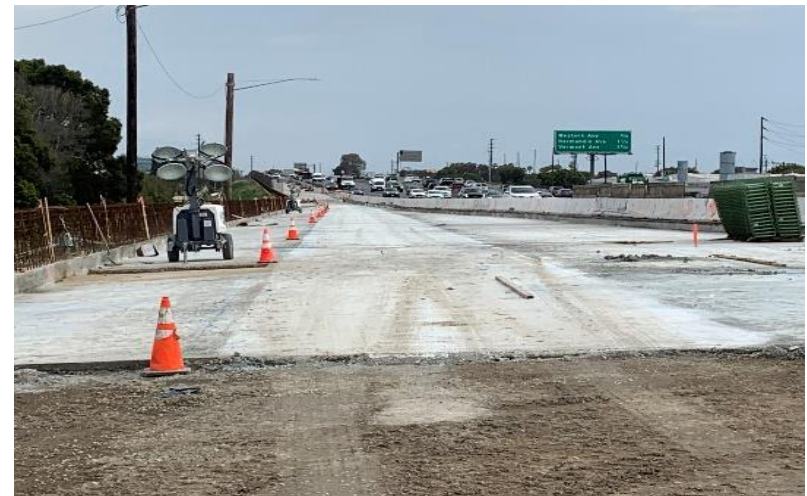
JPCP (Ramp Termini), LCB Paving for NB 405 Crenshaw Blvd off ramp
