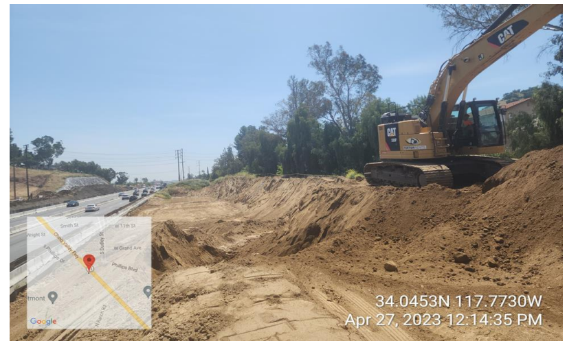
Excavation along southbound roadway
