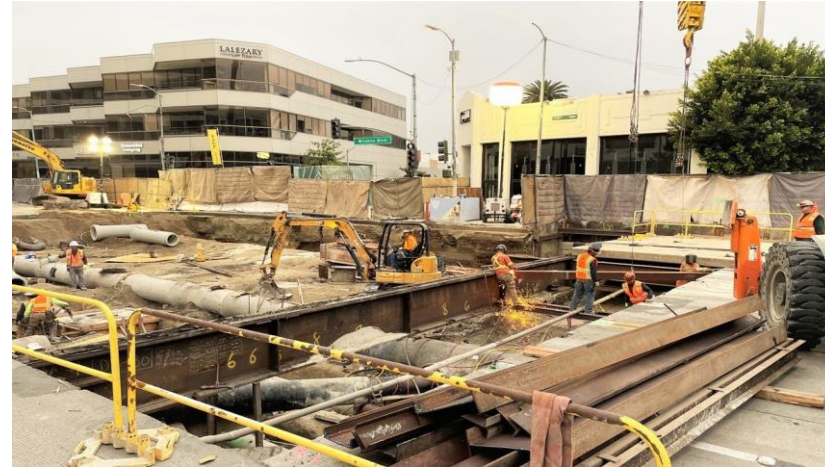
Wilshire/La Cienega Deck Removal/Street Restoration
