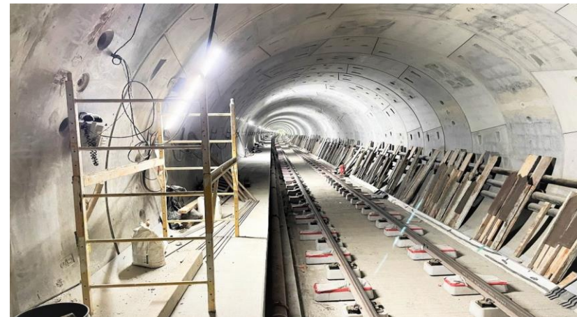
Reach 3 Tunnel (Fairfax to La Cienega) Direct Fixation Blocks and Track Installation
