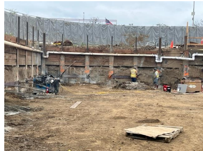
Westwood/VA Station: Tiebacks Installation– North & West Walls
