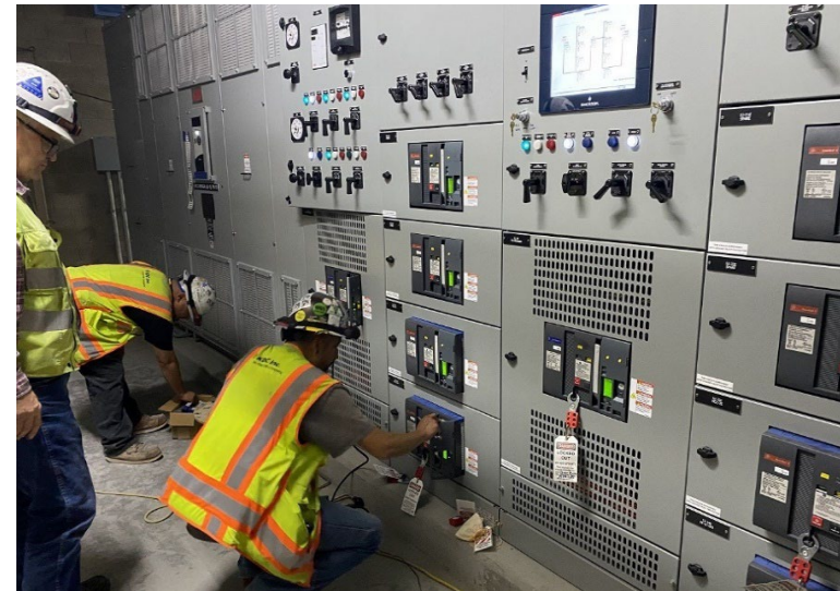
Wilshire/La Cienega Station LFAT Testing
