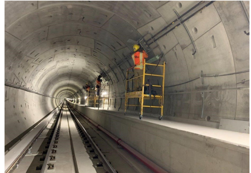
Reach 1 Tunnel Cable Installation
