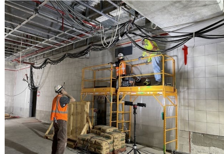
Wilshire/Fairfax Station Porcelain Tile Installation
