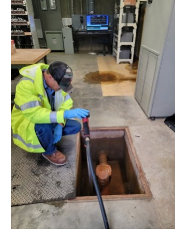
Clogged drain cleared in 90 min.
