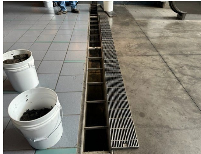
Interior station cleanup to remove debris
