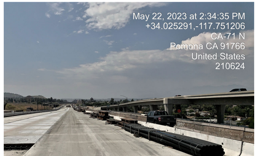
JPCP paving in the median
