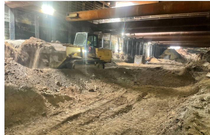
Westwood/UCLA Station: Excavation at Wilshire Blvd
