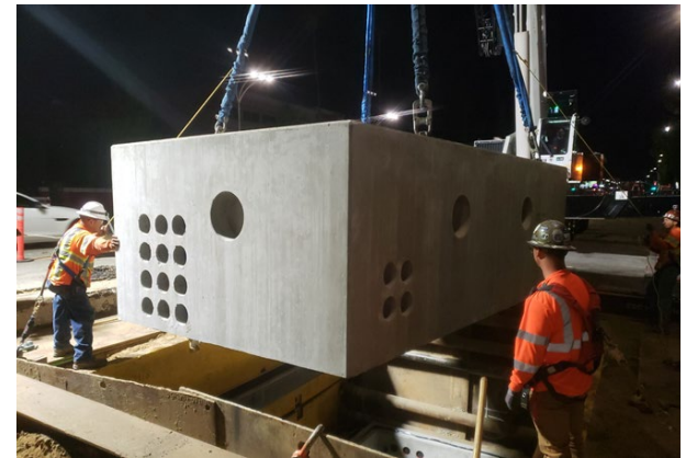
Installation of 1 of 4 vaults by W.A. Rasic on Van Nuys Blvd, between Vanowen and Vose.
