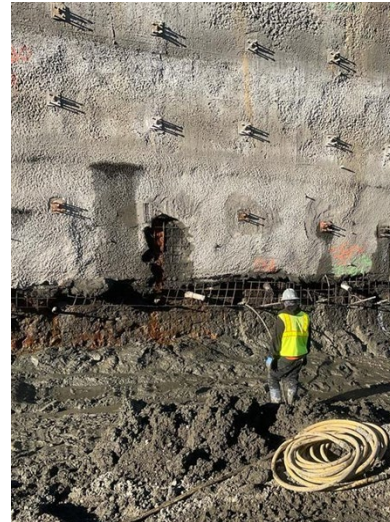
Grouting at Retaining Wall 2461 after March rain storm
