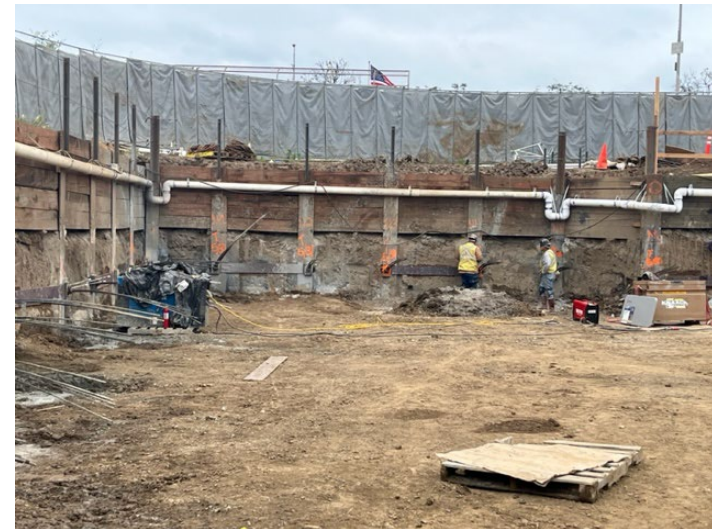
Westwood/VA Station: Tiebacks Installation– North & West Walls
