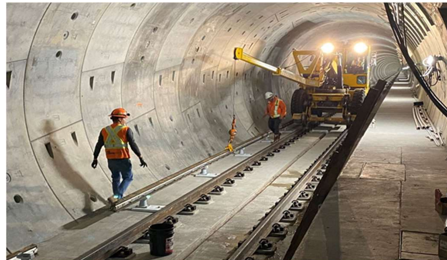
Reach 1 Tunnel (Western to La Brea) Contact Rail Installation
