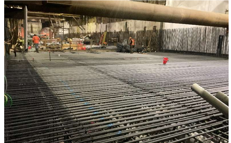
Century City Constellation Station - Top Mat Rebar
