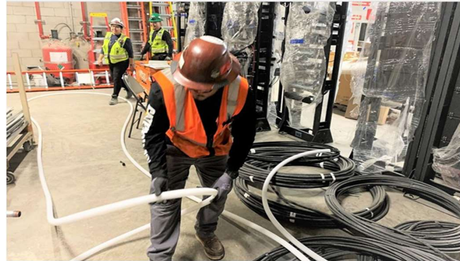
Wilshire/La Brea Communications Cable Installation
