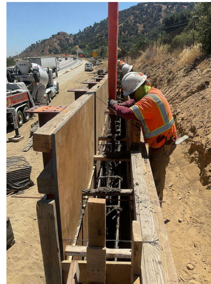
Pouring concrete at Retaining Wall 2461
