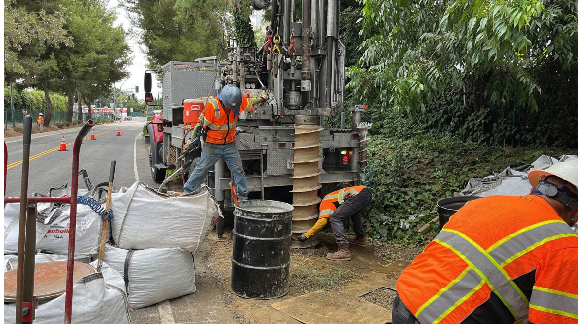
Geotech Deep Infiltration Testing
