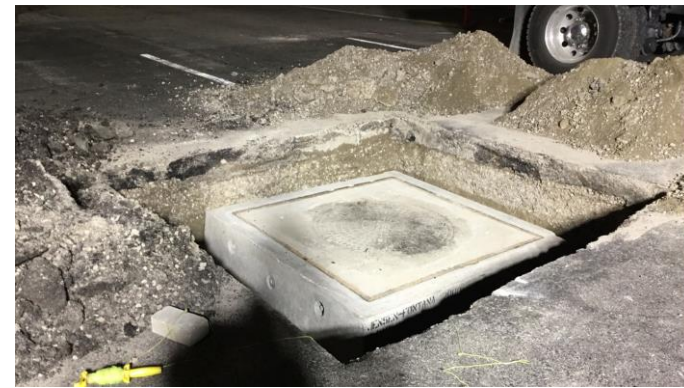
C1220 Manhole Installation
