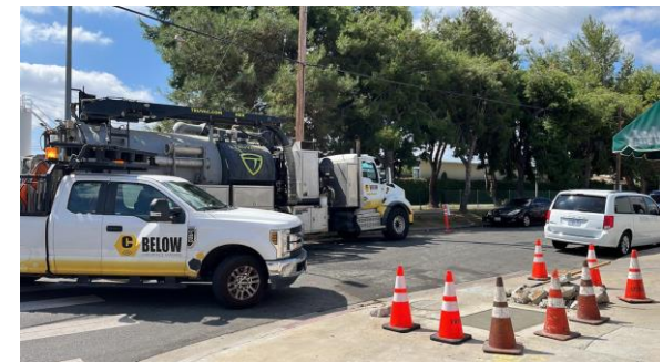
Sidewalk Panel Restoration on Bessemer St
