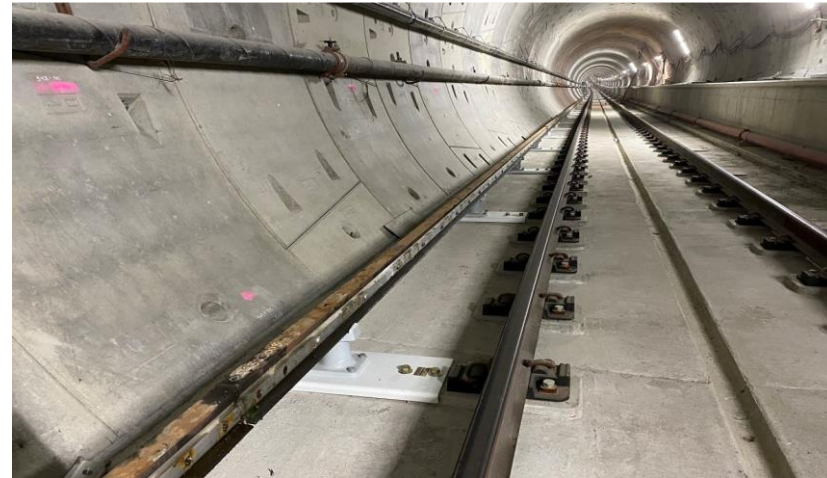
Reach 3 Tunnel (Fairfax to La Cienega)
