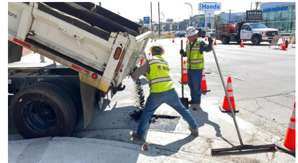
Potholing Restoration on Aetna St
