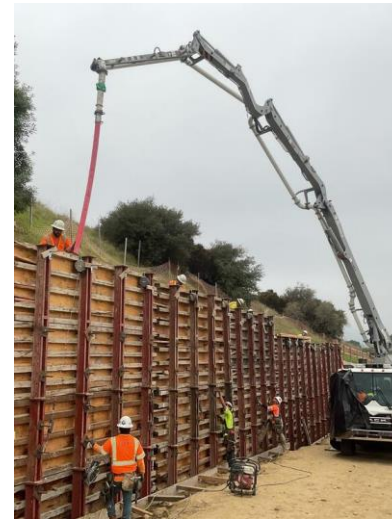
Pouring concrete at Retaining Wall 2461
