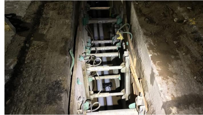
C1220 Ductbank Installation
