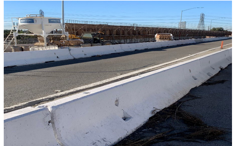
SB 405 Crenshaw Blvd off ramp (SW #815)
