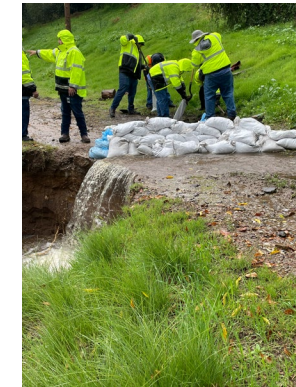
Diverting water from tracks
