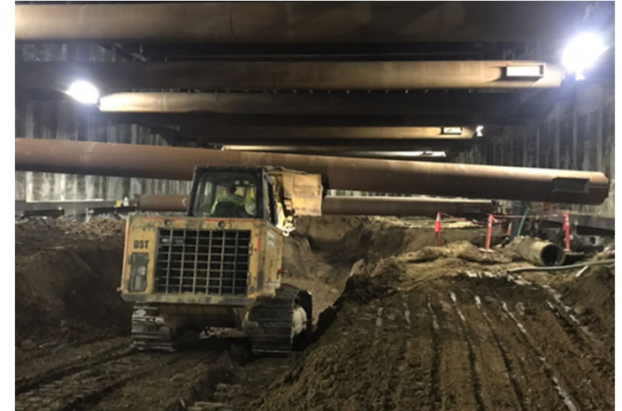
Westwood/UCLA Station: Placement of BL3 Strut
