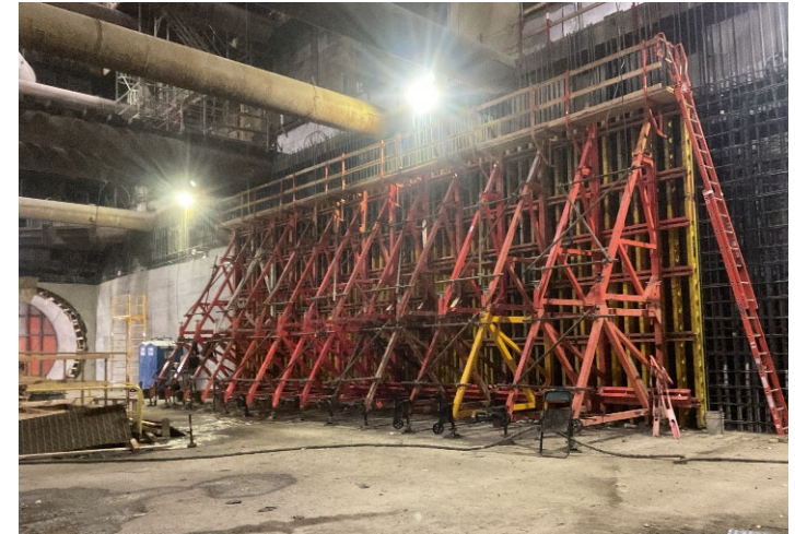
Century City Constellation Station - Concrete Placement
