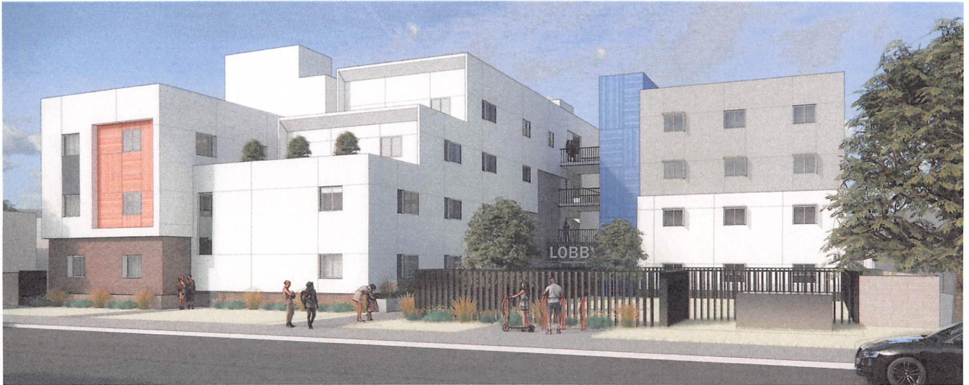
View from Mathews Street facing east
