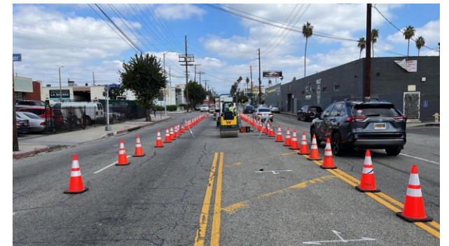
Pothole Restoration on Kester Ave
