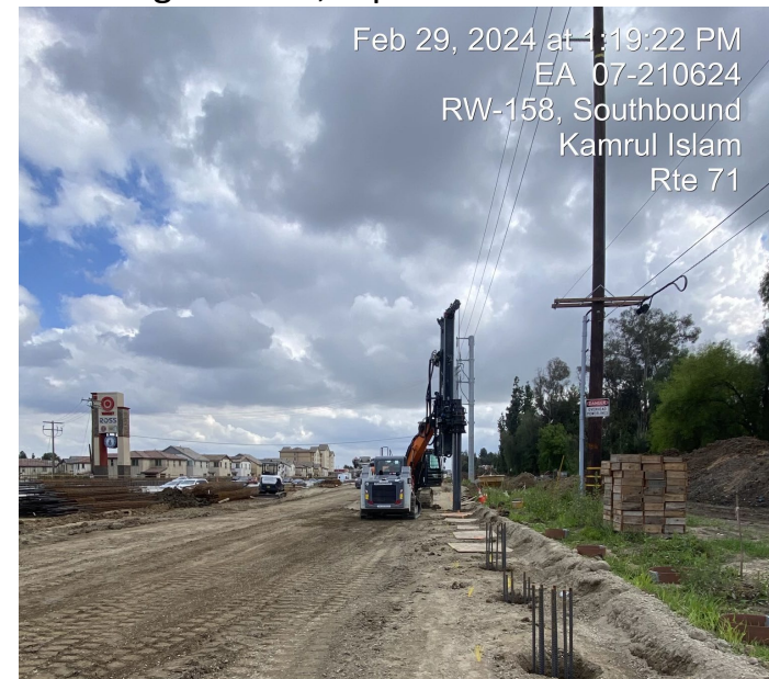
SR-71 SB, SW158 CIDH pile construction.
