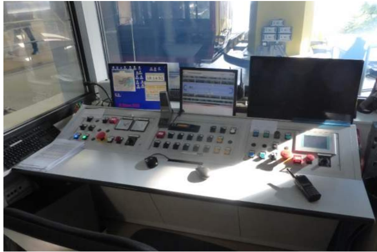
Image 46 – Operator Control Panel
