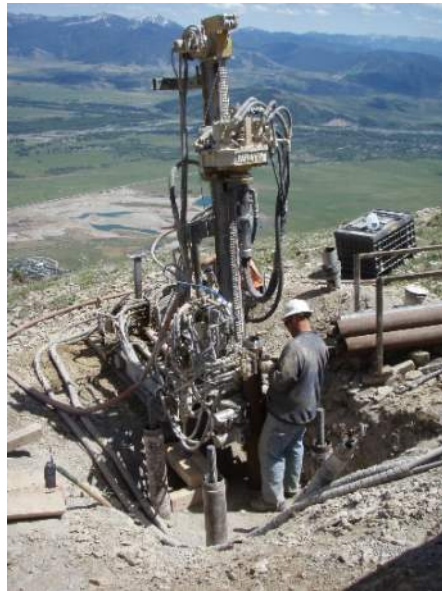
Image 15 – Example of low-impact micropile foundation construction.
