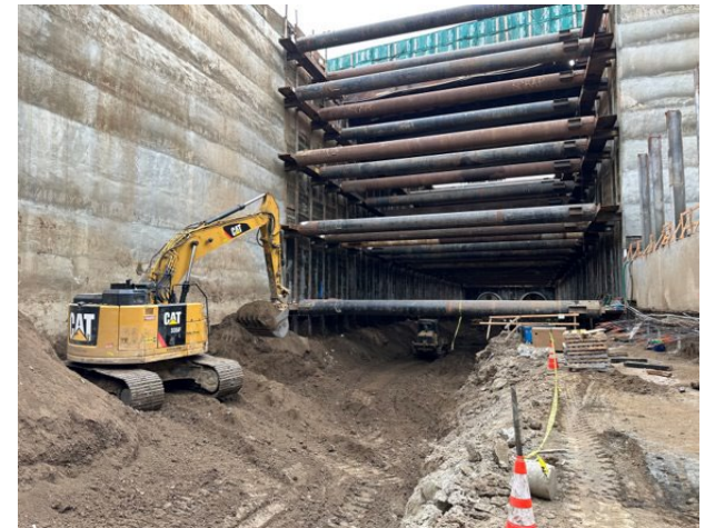
Westwood/VA Hospital Station: Excavation in Station Box
