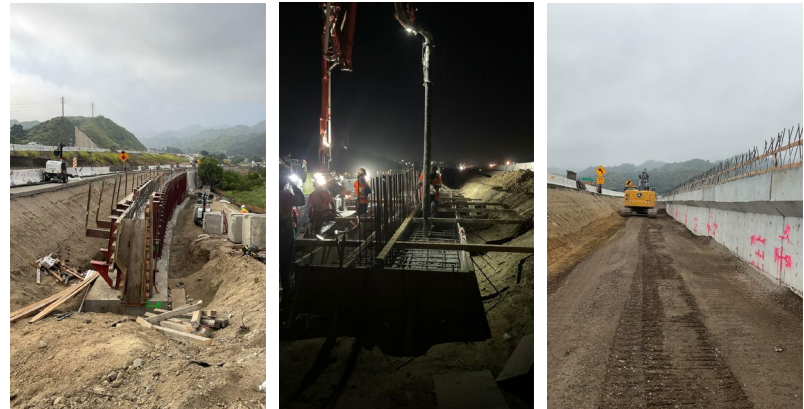
On-going work at Retaining Wall 2577
