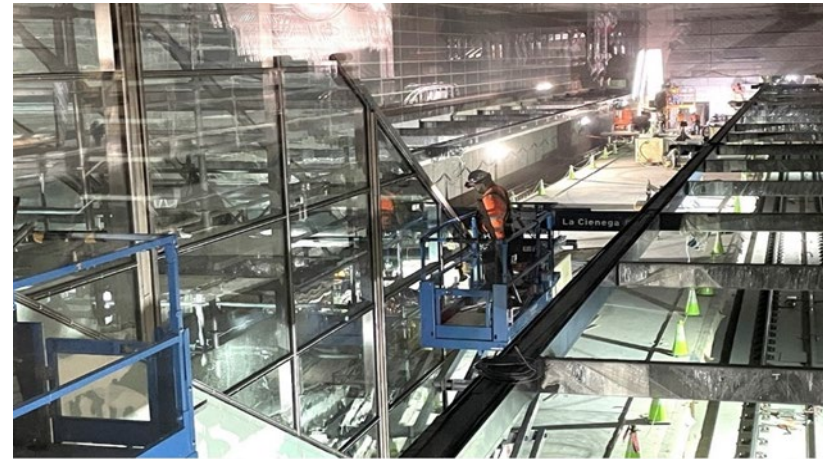
Wilshire/Fairfax Station Smoke Enclosure Glass Installation
