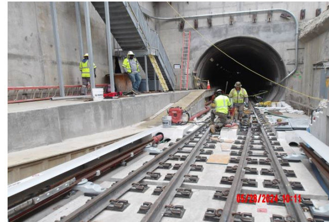
AL Portal work
