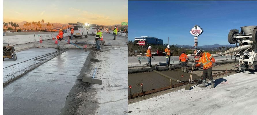
Placement of Lean Concrete Base (LCB) in the median
