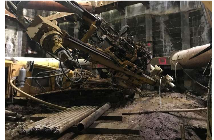
Westwood/UCLA Station: Soil Nail Operation at the West End Wall
