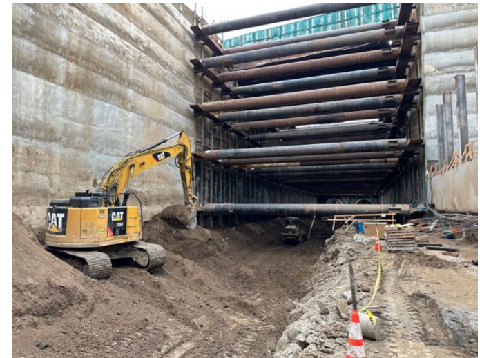
Westwood/VA Hospital Station: Excavation in Station Box
