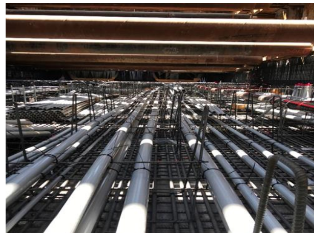
Westwood/VA Hospital Station: Traction Power Conduit Install (Looking West)
