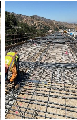
Gavin Canyon Bridge Deck Rebar Install
