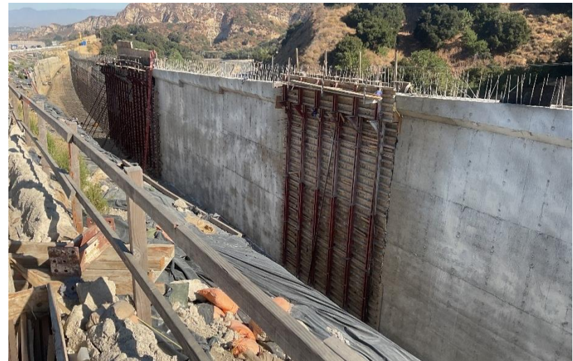
Retaining Wall 2460 formwork installation
