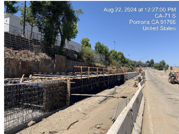
SB-71 DS 16-1, RCB construction progress.
