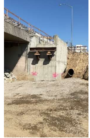
Castaic Creek Bridge Abutment 4 Complete
