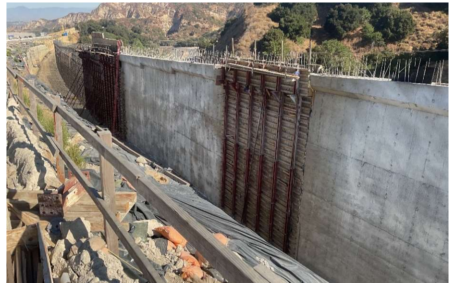
Retaining Wall 2460 formwork installation
