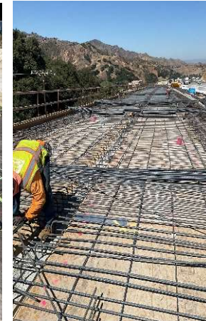
Gavin Canyon Bridge Deck Rebar Install
