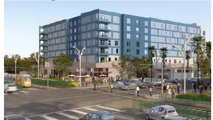
View looking southeast towards the Metro Site
