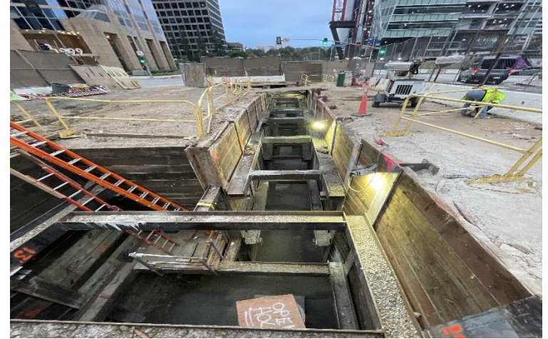
Century City Station Backfill Along Avenue of the Stars
