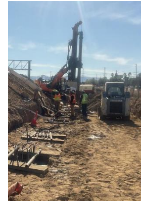
Wall 986 Installation of 24IN CIDH Piling
