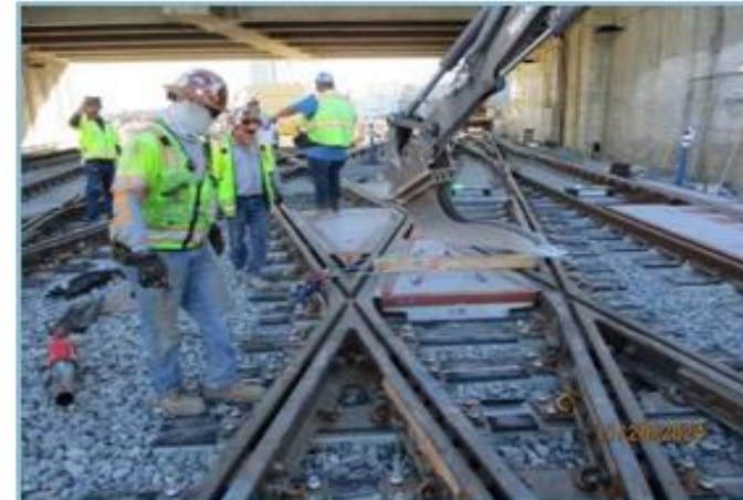
Crossing Panel Installation
