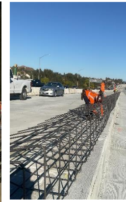
Median Barrier Rebar Installation
