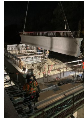
Set Girders at Rye Canyon Bridge
