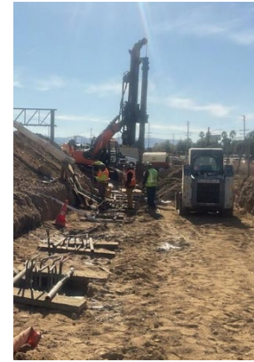
Wall 986 Installation of 24IN CIDH Piling
