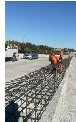
Median Barrier Rebar Installation
