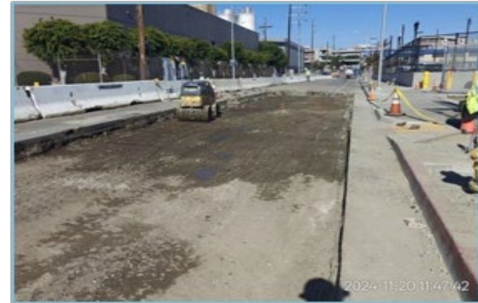
Center Street Reconstruction
