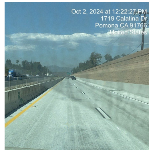
NB-71, completed stage 1 roadway.
