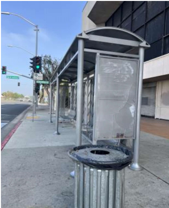
Picture 9 - Hawthorne & Broadway (Broken Plexiglass)
