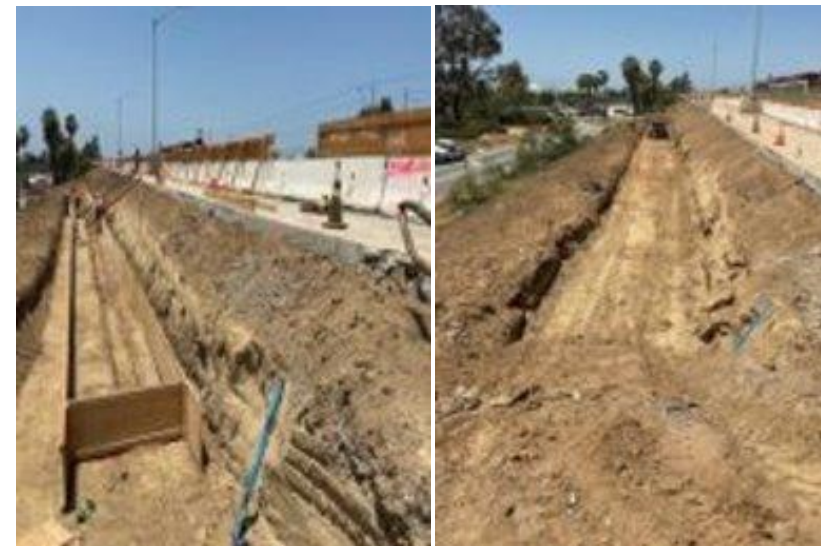
RW 245 Forming Footing
