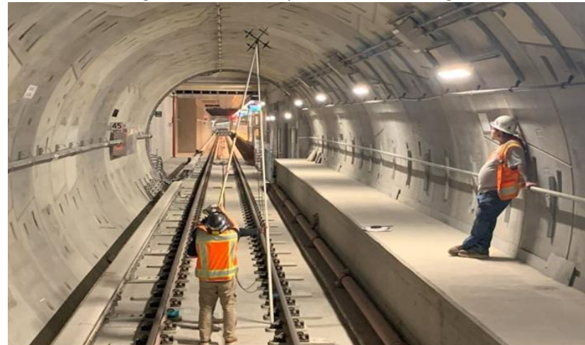
Reach 4 Tunnel (Tail Track)
